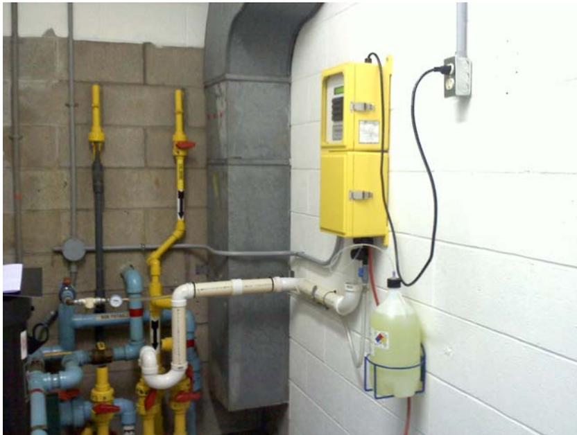
Figure 1. Online Phosphate Analyzer Installation
