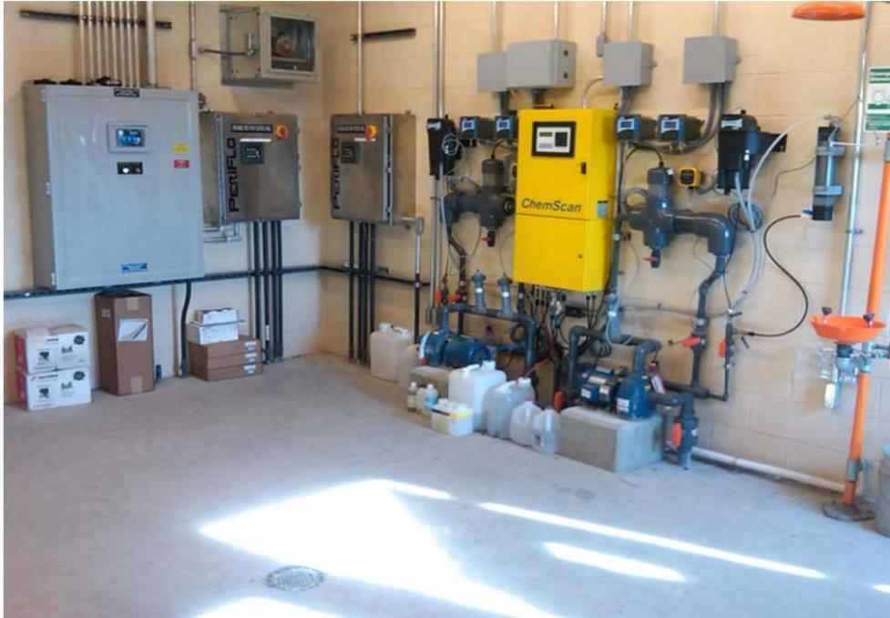
Figure 6. Online Analyzer with Multiple Sample Channel and Multiple Parameters
